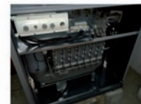
Caldera condensación Wolf. Control de calderas "Improved management by Solvis"
